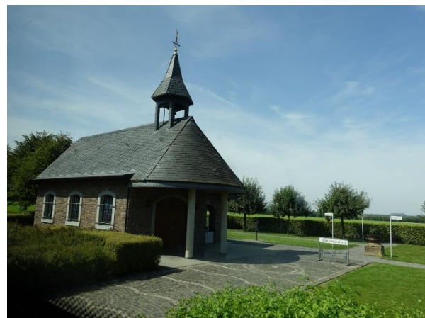
Figure 27: Memorial Chapel in Eschweiler
