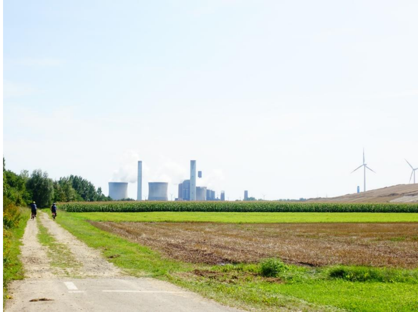
Figure 22: A coal-fired power plant (left) and a wind farm (right) in Eschweiler
